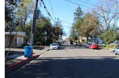
Streetscape: View down Second Street shows a typical Neighborhood classified street, with two unmarked travel lanes, street parking, and sidewalks. Also shows the utility poles and lines that cross the street.
