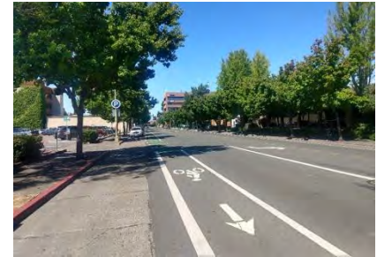
Streetscape: View looking down Third Street shows a well-landscaped streetscape with on-street parking and painted bike lanes.
