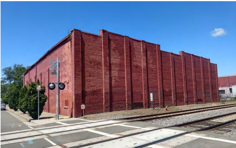
View from West Eighth Street, the red brick façade reflects the historic character of the site and holds the potential for restoration.
