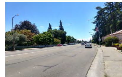
Streetscape: View looking south from Sonoma Avenue, the wide width of the roadway and lack of continuous trees and building frontage give the street an unfinished appearance.
