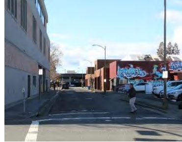
Streetscape: Parking lots, blank building sides, and graffiti negatively affect the pedestrian experience. Looking down Ross Street from Mendocino Avenue.
