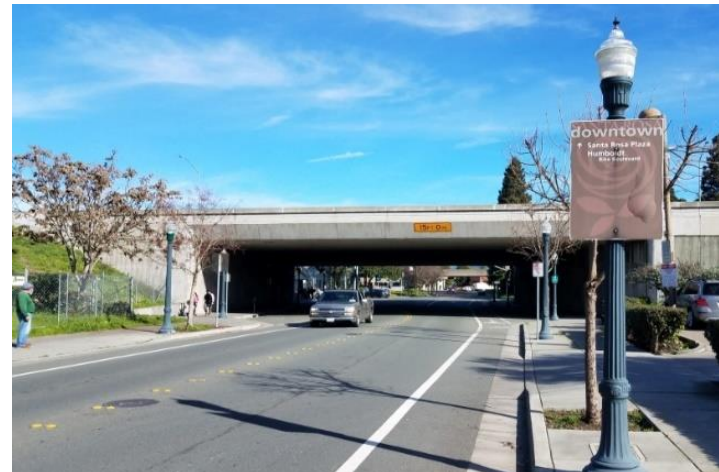
Sixth Street underpass completed in 2013
